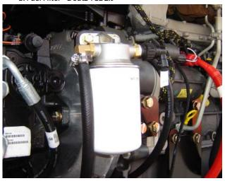
Lube Point(s) - Replaceable Element Interval - Every year or 500 hours of operation
